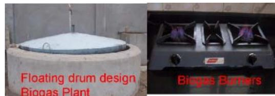
a restaurant near to the house and food waste from this restaurant is put in the biogas plant. Capacity of the biogas is 8 CUM per day, which is too high and can support 8 families like ours.
